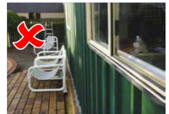
Windows that provide easy access to the pool area must be fixed permanently closed.
