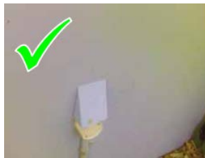
A power outlet has been shielded appropriately.
