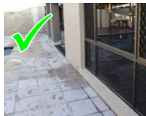
These windows have fixed security screens
