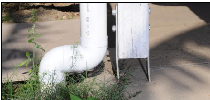
Inspect post brackets for bending or stressing
