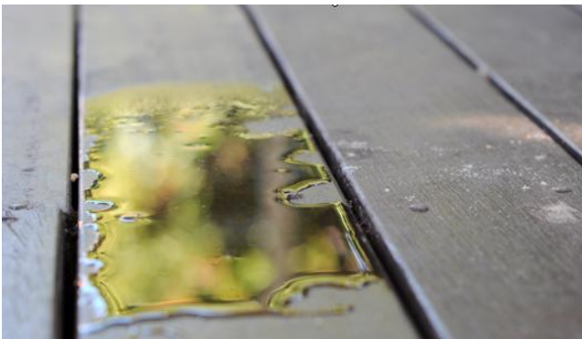
Water left on timber can cause fixings to deteriorate and rust
