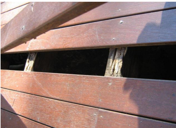
Removing this decking board has revealed a decayed joist
