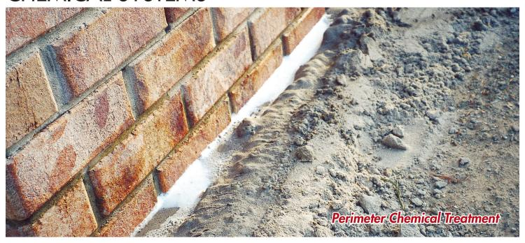
Chemical deterrent systems are normally used in conjunction with slab-on-ground construction. Traditional chemical treatments incorporate a chemical reticulation system under the slab and around the perimeter of the building.
