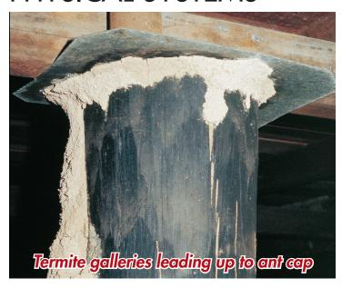
Until recently, physical systems have been restricted mainly to suspended floor construction (e.g.houses built on stumps). The traditional physical system is the ant cap. Ant caps are placed on the tops of stumps and piers etc. Ant caps do not prevent termites from getting into the building, they merely act as a barrier to concealed entry and encourage the termites into the open where they can be noticed during inspections.
