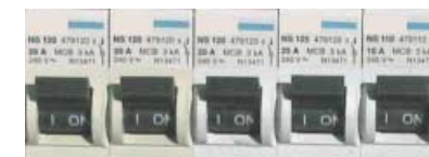
(EXAMPLE OF CIRCUIT BREAKERS)
