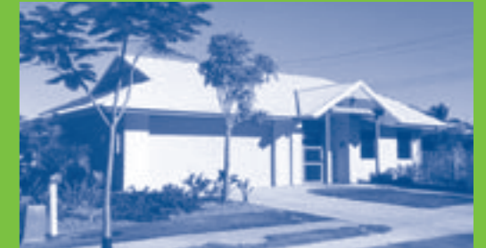
above: Research House, Rockhampton. Designed by the Queensland Department of Housing and the Department of Public Works.
