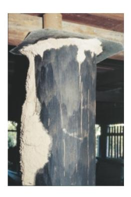
Until recently, physical barriers have been restricted mainly to suspended floor construction (eg houses built on stumps). The traditional physical barrier is the ant cap. Ant caps are used primarily on elevated houses and are placed on the tops of stumps, piers etc.
