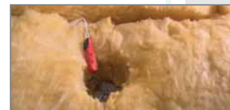
Clearance of 50mm around downlight
