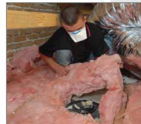
Clearance of 50mm around downlight
