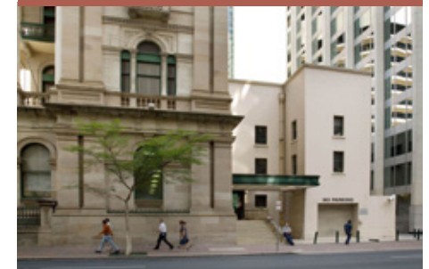
Site prior to development, National Australia Bank, Brisbane, QHR 600153 Photo: Riddel Architecture
