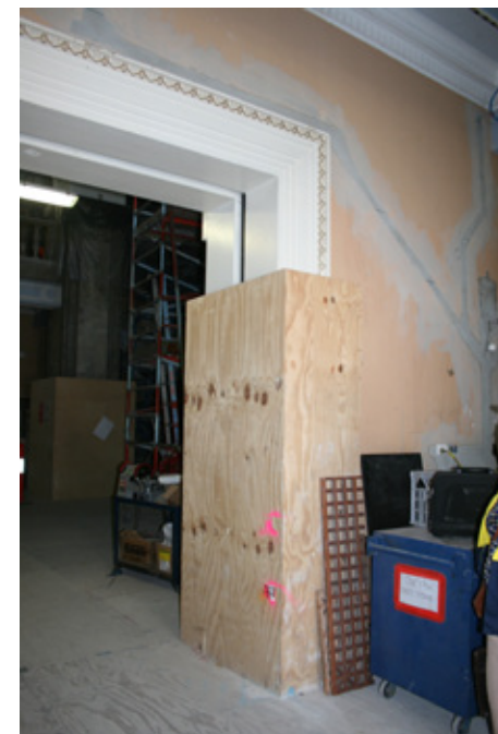
Protective plywood covering installed over door reveals (front right of photo) and marble columns (back left of photo) during restoration of Brisbane City Hall, Brisbane, QHR 600065
