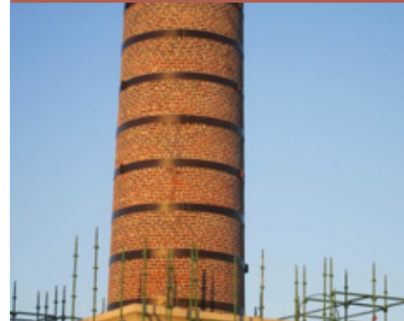
Iron banding on Ross River meatworks chimney, Idalia, QHR 602719 Photo: Townsville City Council
