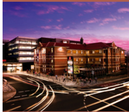
'The Barracks', Petrie Terrace Police Depot (former), Petrie Terrace, QHR 601894 Photo: QM Properties and Property Solutions
