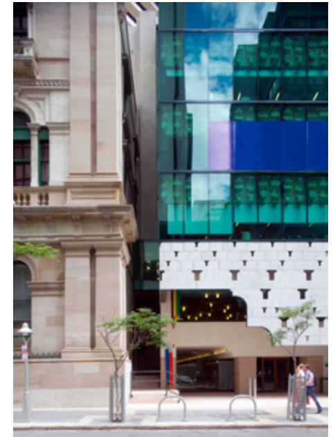
Close up of extension to National Australia Bank, Brisbane, QHR 600153 Photo: Jon Linkins
