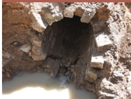
Wheat Creek Culvert during excavation, Brisbane, QHR 602218
