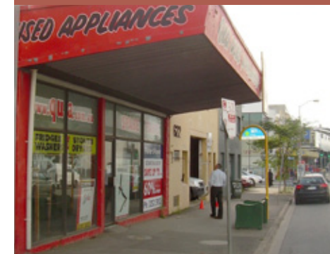
Before restoration, West's furniture showroom (former), Fortitude Valley Photo: Riddel Architecture
