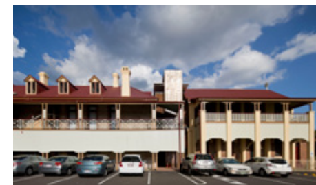
New lift shaft in the gap between buildings at former convent, St Mary's Roman Catholic Precinct, QHR 600577 Photo: Angus Martin
