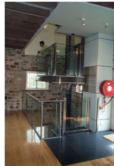
Platform lift, Commissariat Store (former), Brisbane, QHR 600176 Photo: Michael Kennedy Architect
