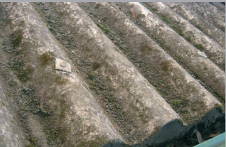
Very poor surfaces of corrugated asbestos cement roof with asbestos debris loose on the roof and in the gutter.
