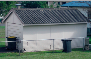
Old Garage: with asbestos cement walls and roof.
