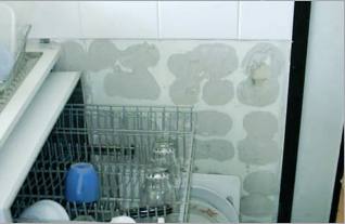
Removal of tiles next to the dishwasher has revealed asbestos cement wall lining.
