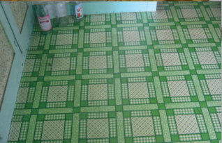
Asbestos backed vinyl in a kitchen.
