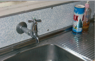
Laminated asbestos cement sheet splash back panel to a sink.
