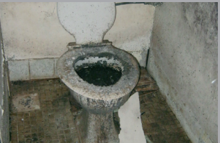
Asbestos cement sheet walls in a toilet.
