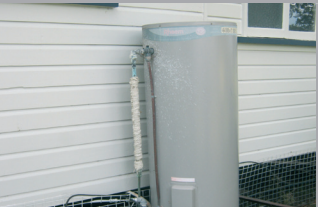
Asbestos woven rope still on a section of hot water pipe leading to a new hot water service unit.
