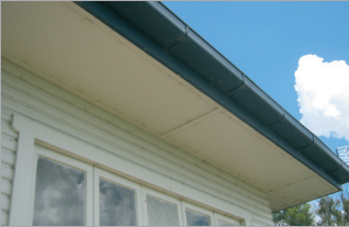
Asbestos cement sheet eaves lining.
