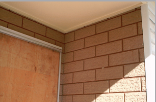
Simulated brick asbestos cement sheet cladding – moulded slices of brick attached to asbestos cement sheeting.
