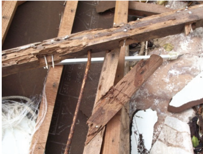
TERMITE ATTACK TO TIMBER
