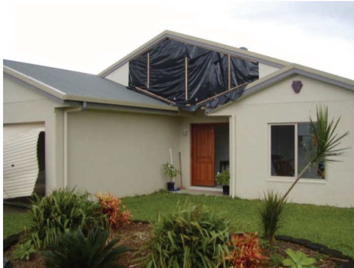
FAILURE OF A GABLE END WALL ALLOWING STRONG WIND AND RAIN WATER INTO THE HOUSE
