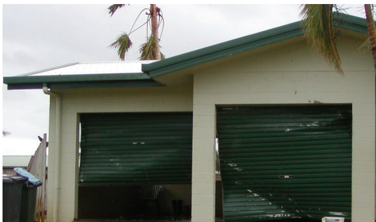
DAMAGE TO GARAGE DOORS.
