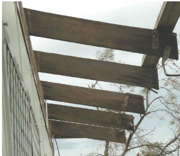
RUSTED BATTEN STRAPS CONTRIBUTING TO ROOF FAILURE
