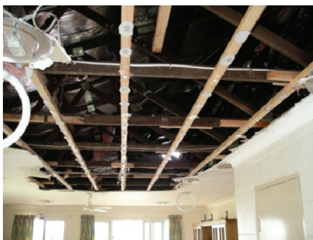
DAMAGE TO CEILING DUE TO WATER INGRESS
