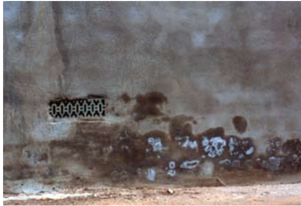
Render showing signs of salt and water.
