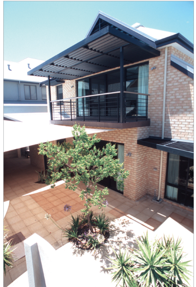
The walls of this house are a combination of double brick and reverse brick veneer.
