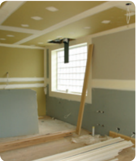
Ensure all fittings and outlets are above possible flood levels. Considering this early on avoids a costly retrofit later on. Photo courtesy of The Courier-Mail.
