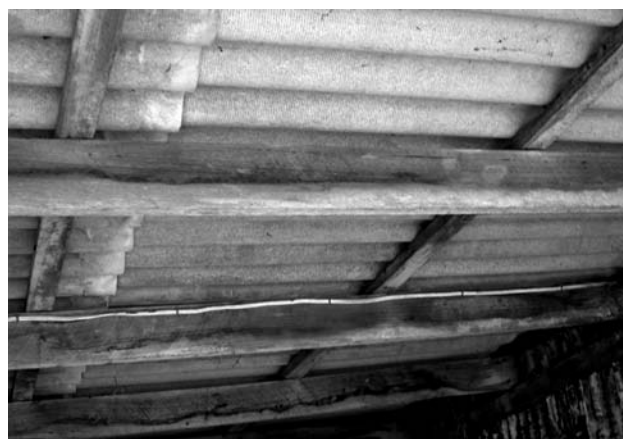
Underside of asbestos cement roof sheeting.
