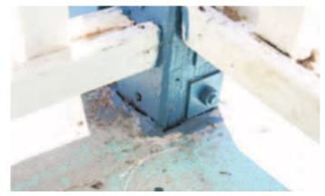
Gaps around base of veranda post allow water ingress into wall cavity
