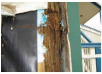
Rotted wall studs below the bearer support joint
