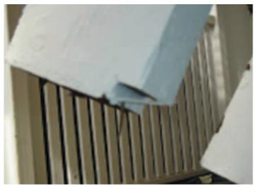
Paint clearly evident inside the cog in the joist
