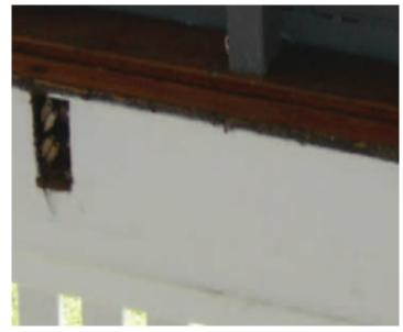
Mud wasp nests in the bearer housing is evidence that a sizeable gap existed where the floor joist  $\cos$  was not fully engaged into the bearer
