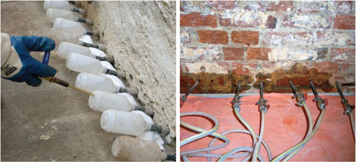
Figure 41 and 42 Chemical impregnation. On the left: the gravity-fed system in which small plastic bottles are filled with a lance. Depending on the nature of the masonry and thickness of the wall the bottles are filled three and sometimes four times. Open holes just above the drilled line are used to indicate extent of penetration. On the right: low-pressure injection in progress on an interior wall from which plaster has been removed. Note the variation in the permeability of the brickwork; the brick on the left is already saturated and the lance is moved on while the central brick slowly fills with fluid.
