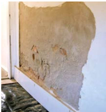
Figure 31 Sacrificial plaster decaying as intended. Plastic sheeting is used to catch the salts and prevent their recycling through the soils and walls.
