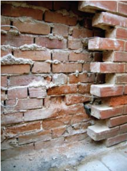
Figure 45 Decay of an inner leaf of brickwork into the cavity. This would not have been discovered had the wall not been opened up for undersetting of the outer leaf. The decay means that evaporation is occurring in the cavity in preference to the interior of the house. Multiple paint coatings or previous repairs of interior plasters with dense impermeable materials may be an explanation. Whatever the cause, the implications of decay occurring where it cannot be seen are profound. The inner leaf must be treated, using one of the methods described in this guide.
