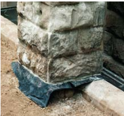
Figure 38 Insertion of a DPC by slot sawing. A mortar joint is sawn out with a chainsaw allowing insertion of DPC sheeting. As salt-laden stone is left above the DPC, the technique must be combined with desalination to be successful.
