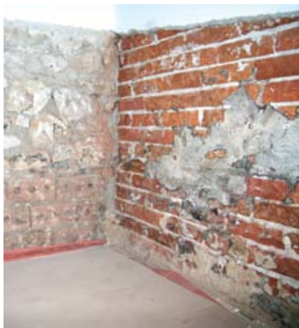
Figure 51 Discoveries on removing plaster from interior walls. On the left, the brick-on-edge is a partial undersetting of the inner part of a solid wall, leaving the outer part untreated — a total waste of effort. On both walls, but more apparent on the right, are remnants of a dense hard cementitious material containing milled iron that was designed to rust and block pores, making it impermeable. Its removal proved extremely difficult.
