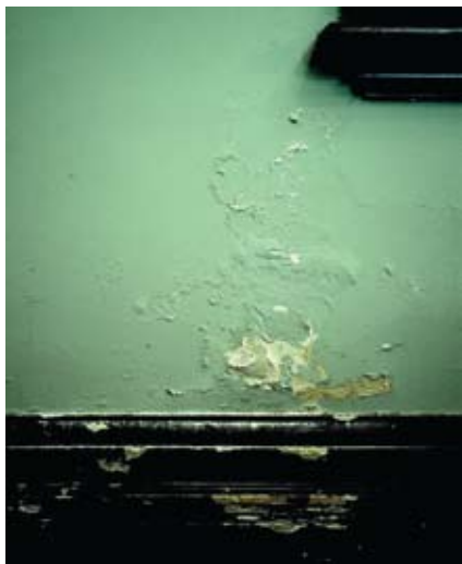
Figure 7 Typical blistering of paintwork and damage to internal plaster due to the combined effects of rising damp and salt attack. The skirting is a cement moulding and also shows salt damage.
