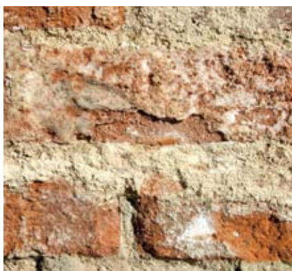
Figure 52 A thick film of salt that crystallised beneath a hard render, which was in turn finished with a high-build (thick) paint coating. For evaporation (and hence salt crystallisation) to occur the render must first have become partially detached from the brickwork. Thermal cycling would then drive air movement, allowing evaporation. The salt was chiselled off and the brickwork poulticed before re-rendering.
