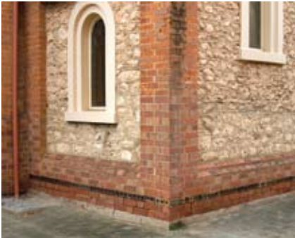
Figure 37 Undersetting from the 1930s. New bricks and stones have been inserted up to a line above the window sill on the left. Bricks below the DPC are visibly damp (see also Figure 10).
