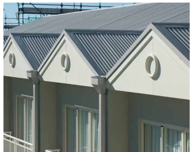
Flashings provide the essential weatherproofing at the edges, and they sharpen the image of the finished job.
