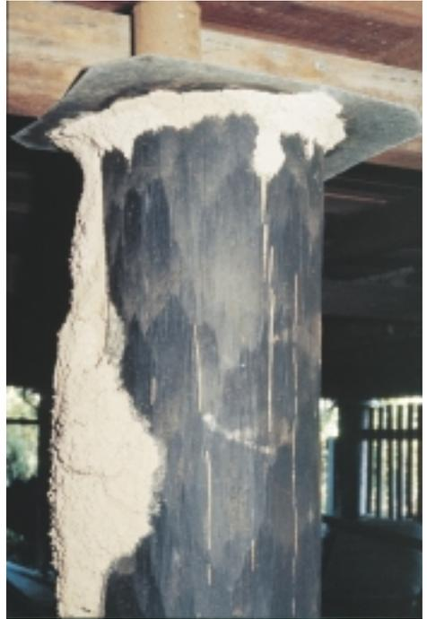
Until recently, physical barriers have been restricted mainly to suspended floor construction (eg houses built on stumps). The traditional physical barrier is the ant cap. Ant caps are used primarily on elevated houses and are placed on the tops of stumps, piers etc.
