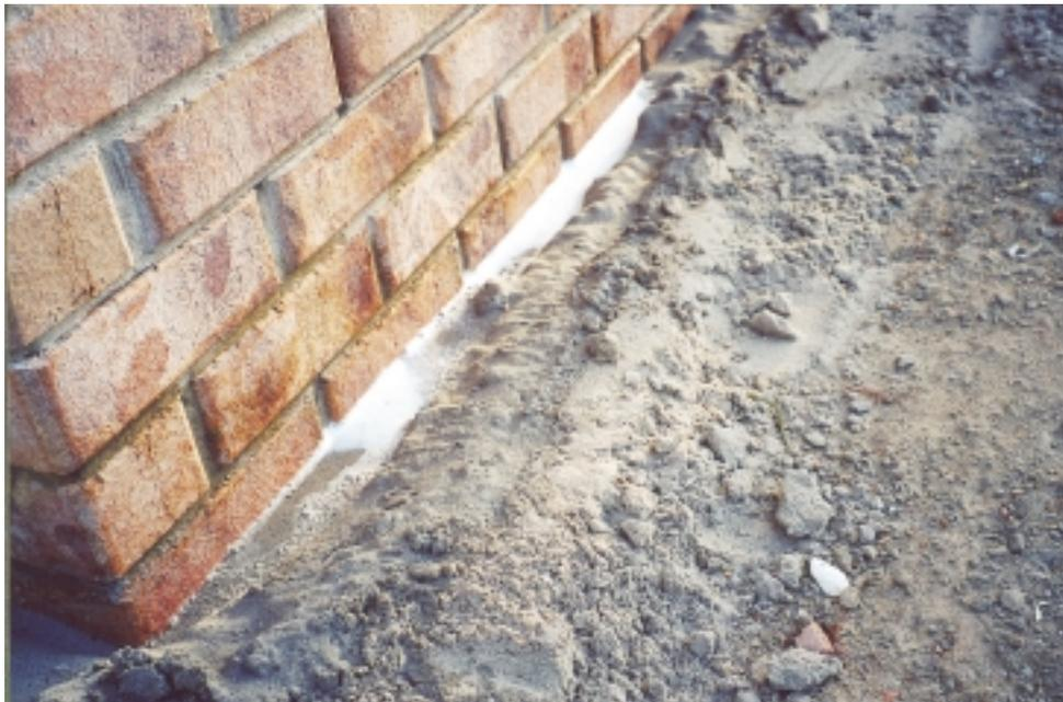
Chemical barriers are normally used in conjunction with slab-on-ground construction. Traditional chemical treatments incorporate a chemical barrier under the slab and around the perimeter of the building.
