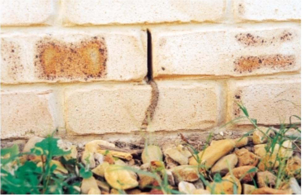
Regardless of the system used, regular inspections by a BSA licensed contractor should be carried out to ensure termites have not crossed (bridged) the barrier. It is recommended that inspections be at intervals not exceeding 12 months.
