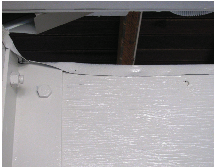
Photo 4: Flashing installed over H3 LVL beam under a deck
