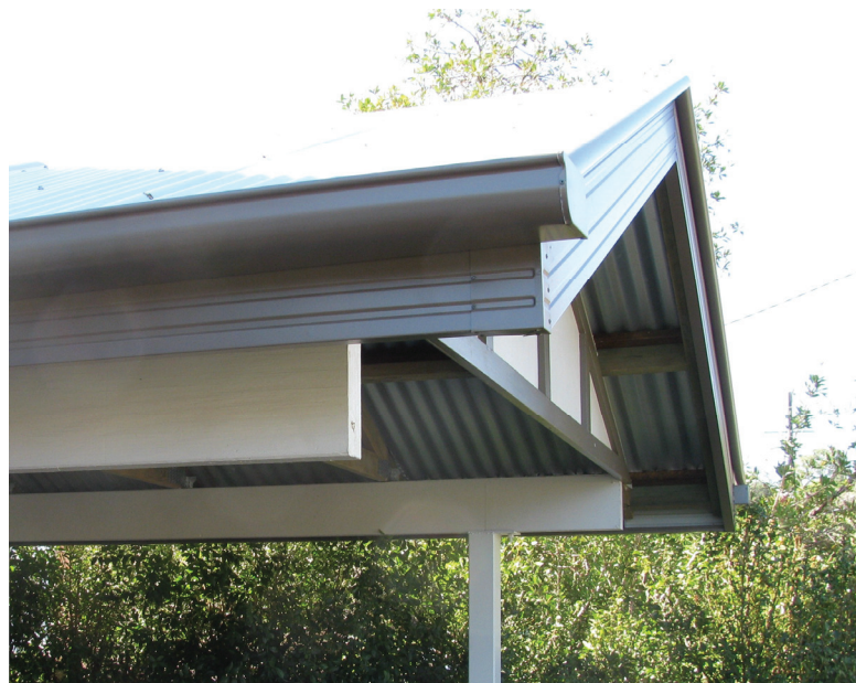
Photo 3: Adequate overhang and quality pale coloured paint system provide good protection to end grain and sun exposure
