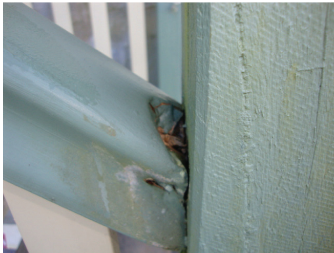
Photo 1: - Avoid premature failure by applying supplementary preservative and oil-based alkyd primers on all cuts, notches, holes etc
