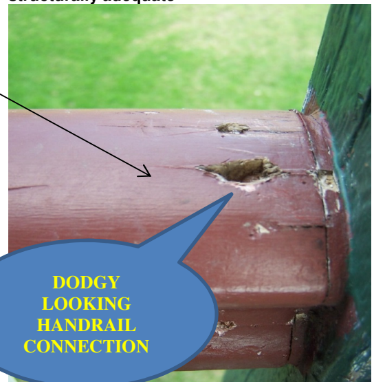
Make sure handrail connections are structurally adequate
