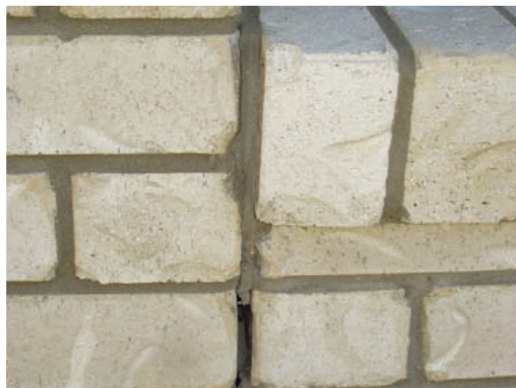
Articulation joint not carried through sill
