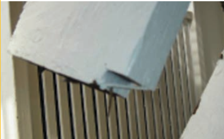
Paint clearly evident inside the cog in the joist.
