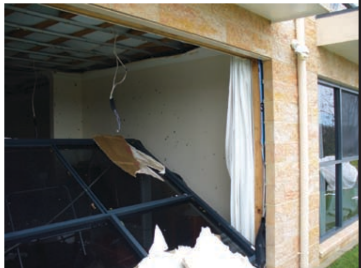
Whole window assembly blown in without breaking the glass
