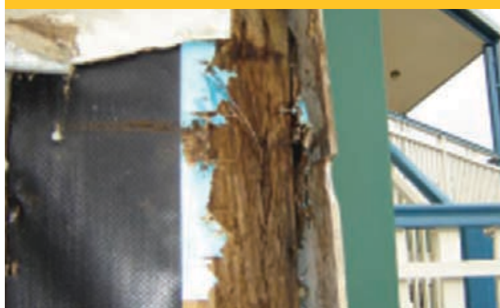
Rotted wall studs below the bearer support joint
