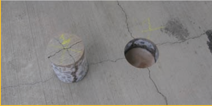
Plastic settlement cracking
