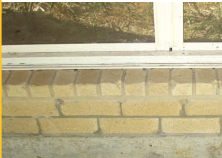
Mortar joint of variable width and significantly exceeding 10mm in places.
