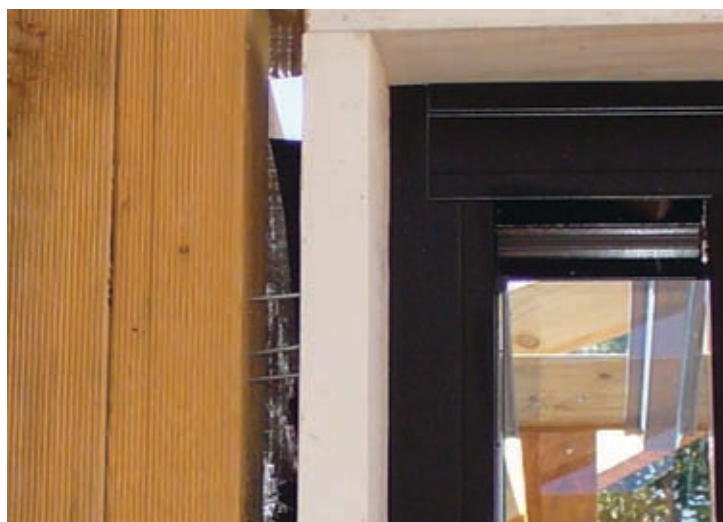
Inadequate fixings - excessive gaps, no packing, nails too short to bridge the gap and securely fix to the frame
