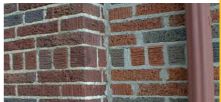
Colour differences in brick work can be a subjective issue
