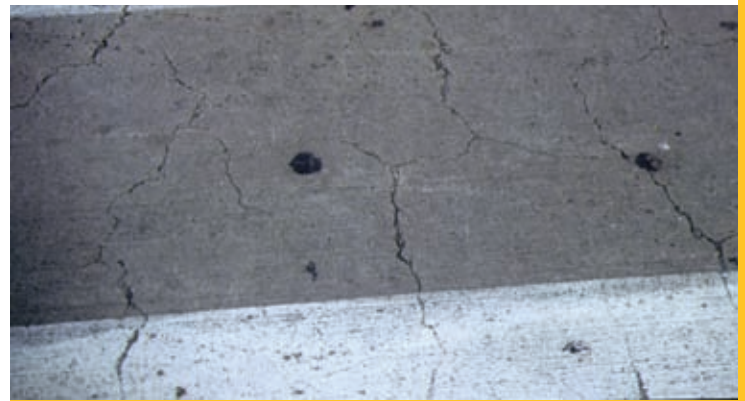
Plastic shrinkage cracking
