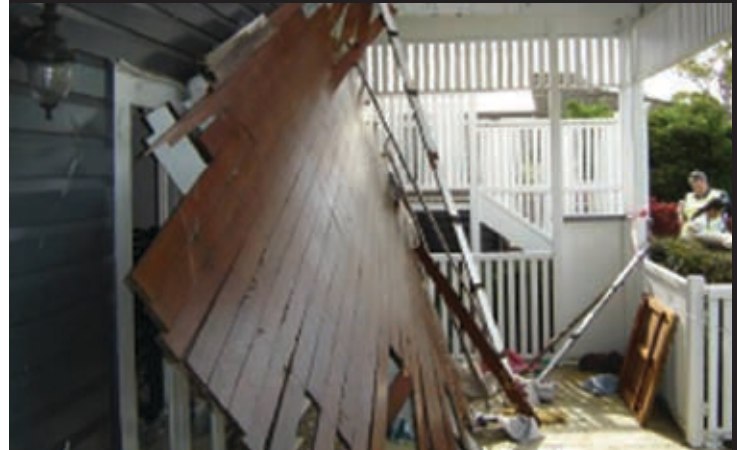
View of collapsed deck
