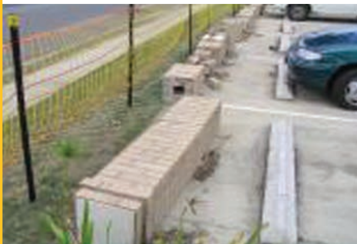
Brick work piers in fencing with no vertical reinforcing
