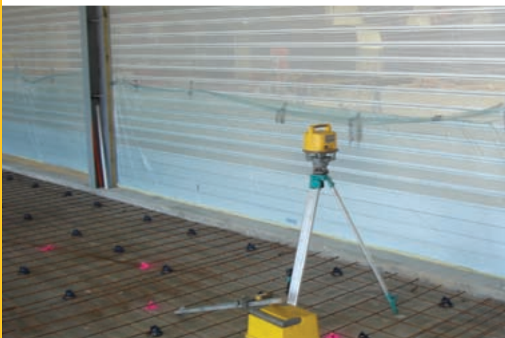
Plastic Film Protection over Roller Grilles
