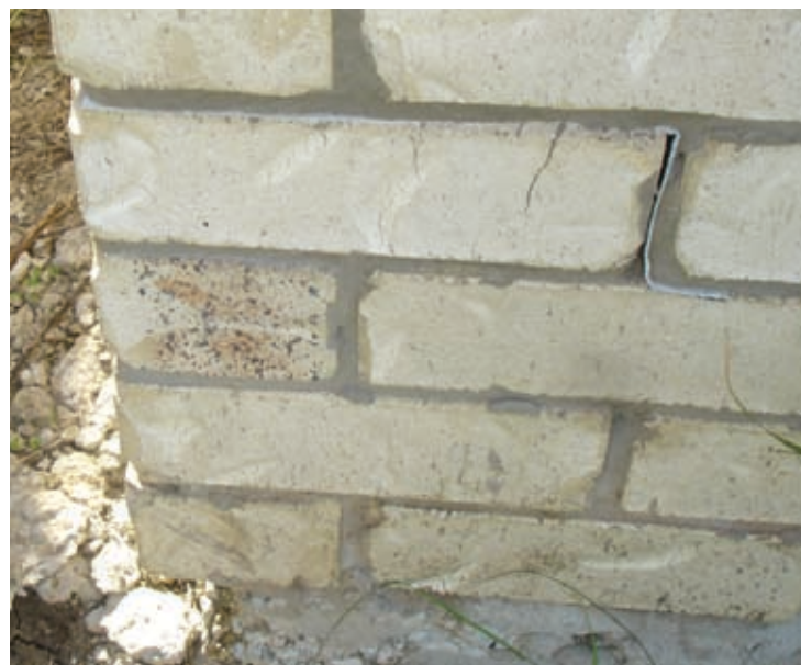
First course significantly overhanging slab edge
