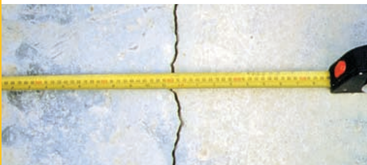
Drying Shrinkage Cracking
