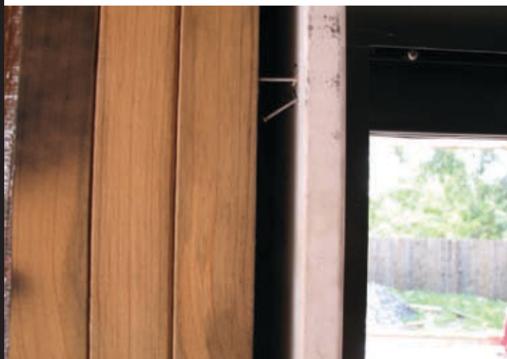
Inadequate fixings - excessive gaps, no packing, nails too short to bridge the gap and securely fix to the frame
