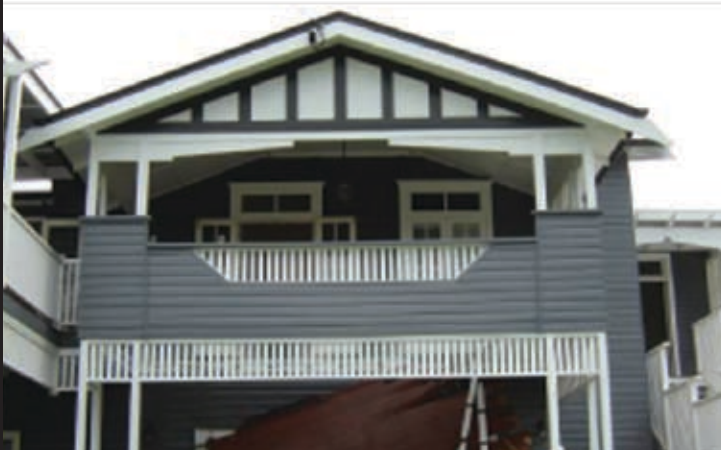
Ascot residence subject to balcony collapse
