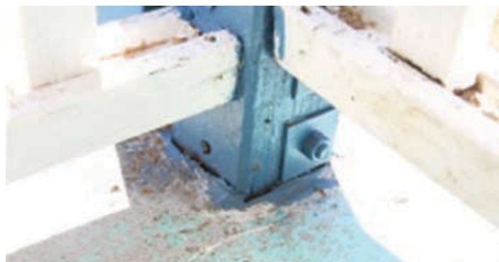
Gaps around base of veranda post allow water ingress into wall cavity
