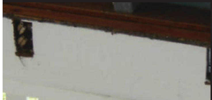
Mud wasp nests in bearer housing is evidence that a sizeable gap existed where the floor joist cog was not fully engaging into bearer.
