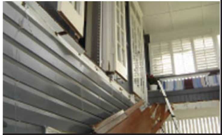
View at internal wall of home external bearer support
