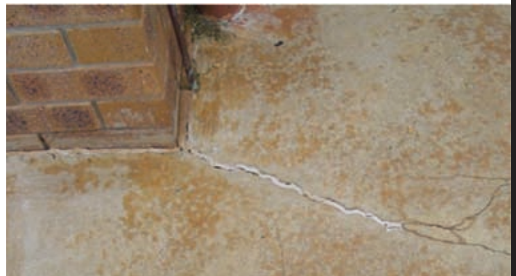
Cracks occurring at change of direction
