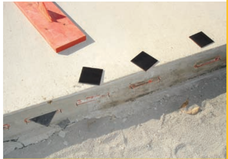
Engineer designed construction joint
