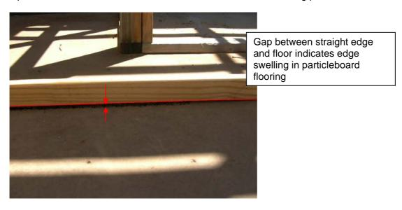
Timber floors on concrete slabs (includes, overlay, T&G on ply or battens, direct fix etc) Remove and replace as it is highly unlikely that an acceptable floor will be able to be obtained from the original floor. Moisture, mud and silt will have become trapped under the floor surface.
