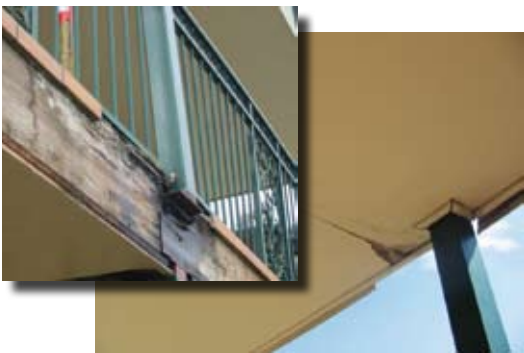
These photographs show a timber bearer of inadequate durability and an inadequate perimeter membrane detail
