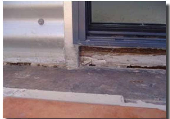
This photograph shows the result of a poorly constructed membrane system that, amongst other things, had inadequate turn up and protection at the junction with external walls and under the door sill.
