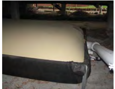
Bladder tank installed under house and full of rainwater
