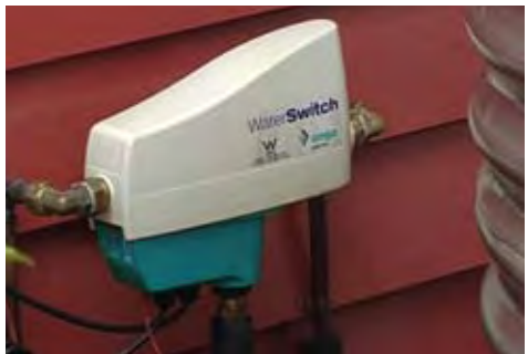
Alternative style of automatic switching device
