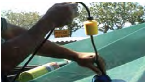
Float switch for Automatic switching device is installed to tank
