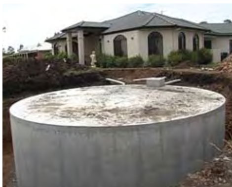
This concrete tank was built on site
