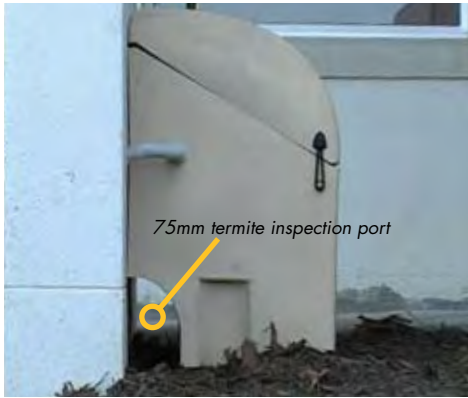
Automatic switching device installed in waterproof cover with in-built 75mm termite inspection port
