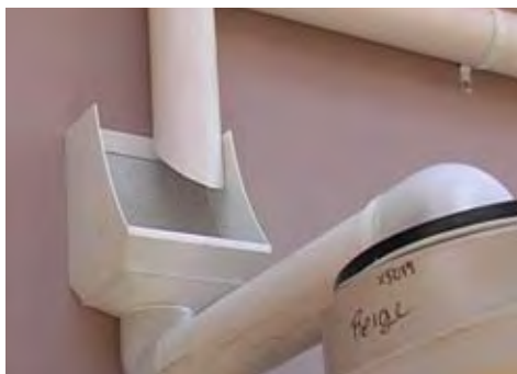
Leaf & debris screen on rainwater head
