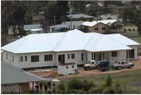
Big roof areas offer the opportunity to collect large quantities of rainwater for domestic use.
