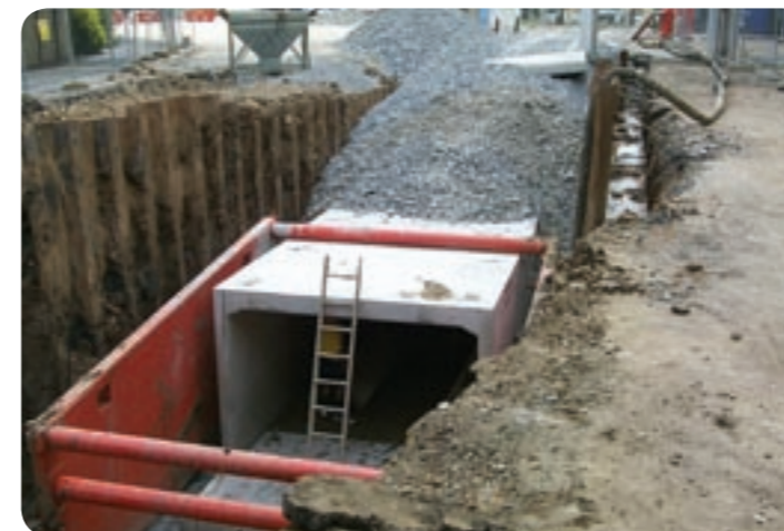
Council invests in mitigation works to minimise flooding in Brisbane.
